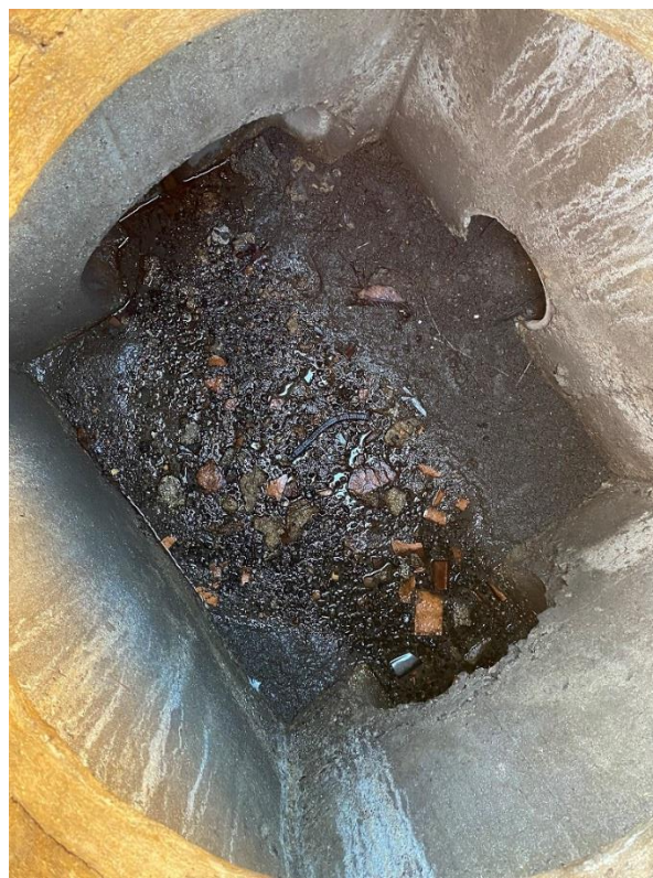
Photo 15-Plot béton Totem 1,30*1,30*0,65m
