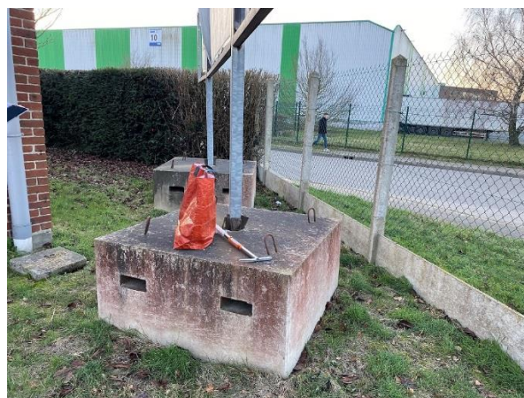
Photo 15-Plot béton Totem 1,30*1,30*0,65m
